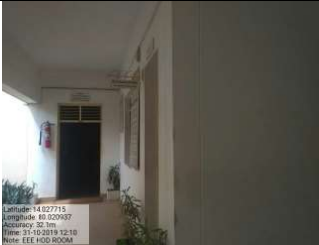
EEE HOD ROOM
